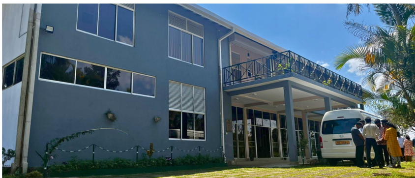
Renovation of District Ministry Centre in South Asia
